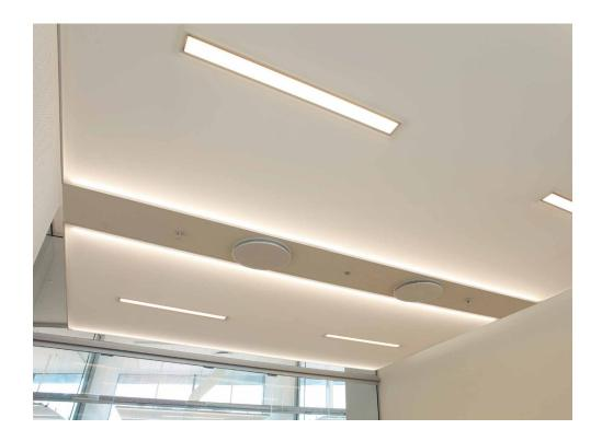
Another CLIPSO advantage is dry installation at room temperature (no odours, no drying time, very little dust or waste), guaranteeing a room ready for use and looking great in next to no time. A process perfectly suited to occupied spaces such as offices. These impressively large lit ceilings are elegant and functional and have enabled the ceiling height to be adjusted whilst creating a more attractive workspace - precisely the client's desired effect!
