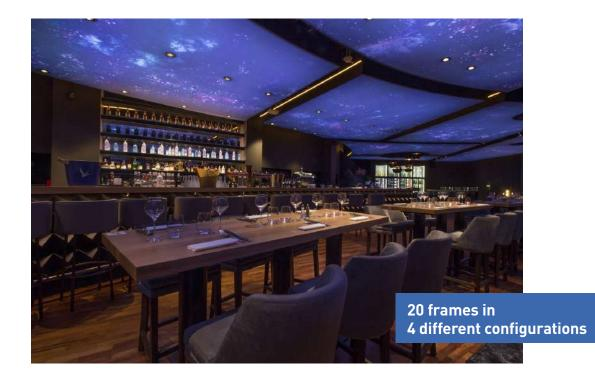
Lowered by almost two meters, the ceiling of the restaurant area has been completely reorganized with XXL acoustic frames. Custom made, the 18 structures in 140 mm thick aluminum profiles were manufactured by the Alsatian company.
