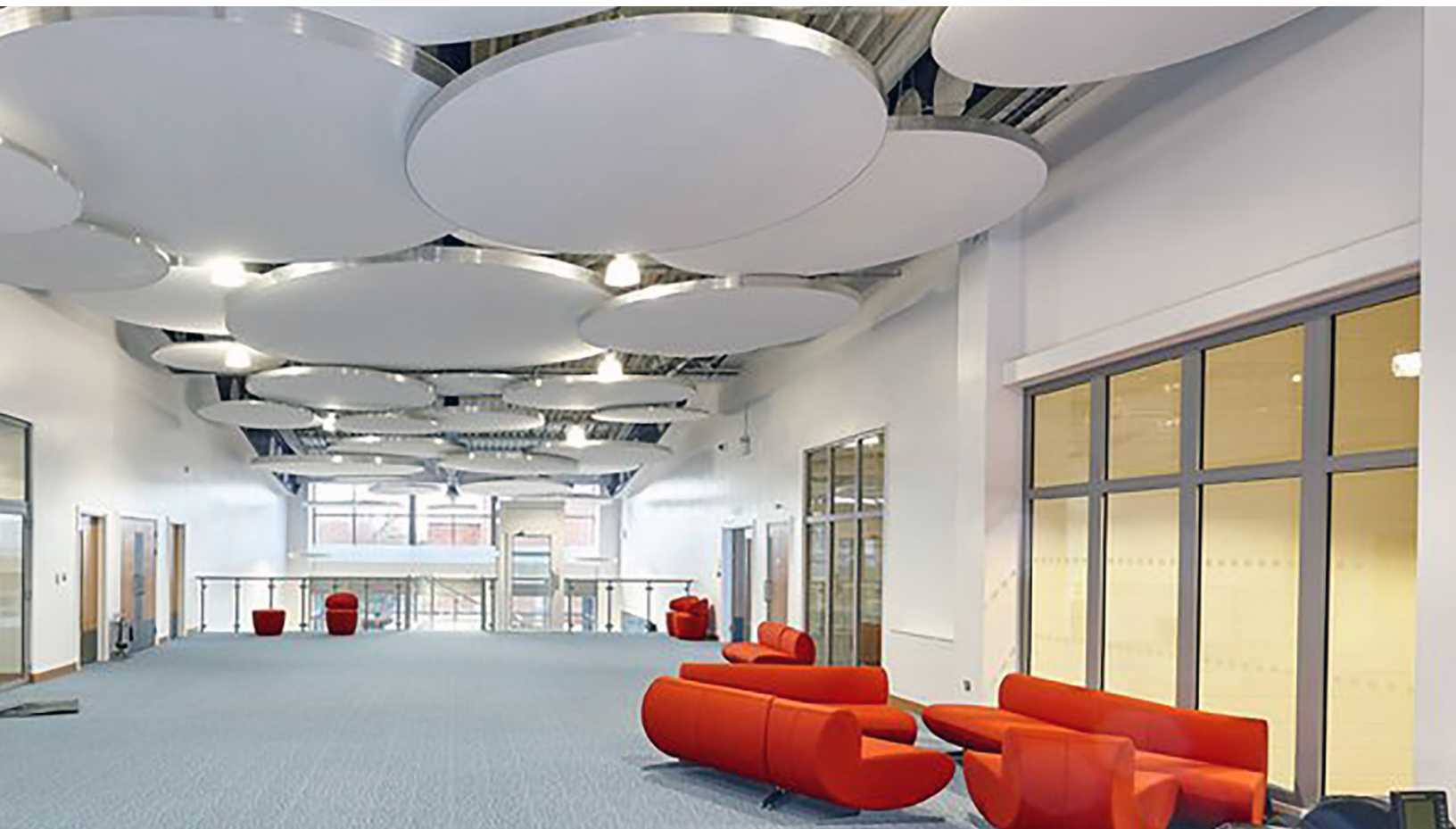
Haberdasher School (UK). 37 circles of varying diameter: from 2.00m to 5.00m. Thickness: 43, 100, 140 mm. White covering and sound absorbent.
