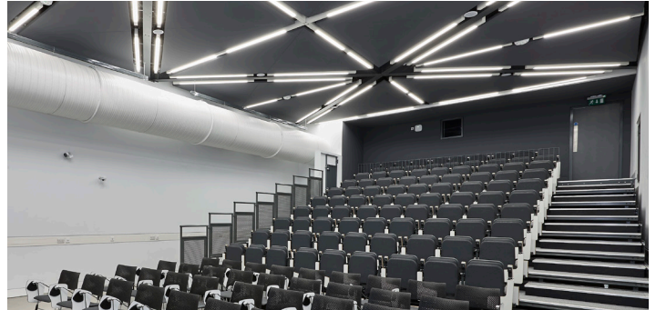
Conference room, Winchester (UK). Triangular acoustic frames. Dim. 3.60 m x 1.30 m x 2.30 m. Thickness 43 mm. Sound absorbent and grey finish. Integrated lighting.
