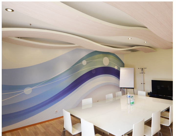
Meeting room, France. "Wave" frame Dim: 5.90 m x 0.40 m. Thickness 43 mm. Material effect print covering.
