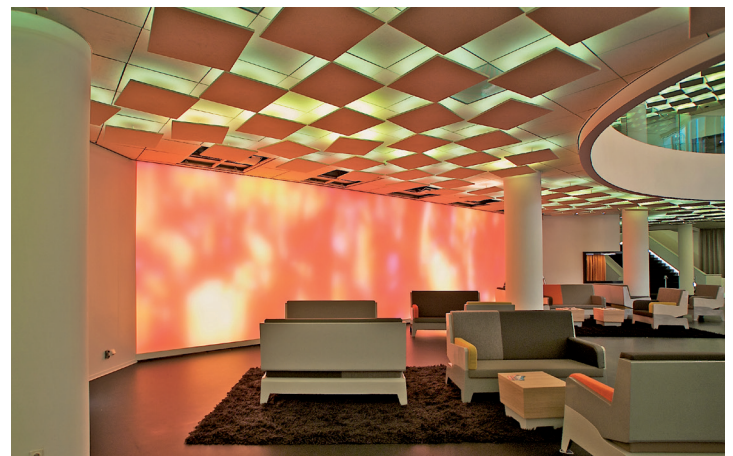
Rest area, Netherlands. Suspended panels. Dim: 0.60 m x 0.60 m. Translucent and colour covering. Integrated lighting.
