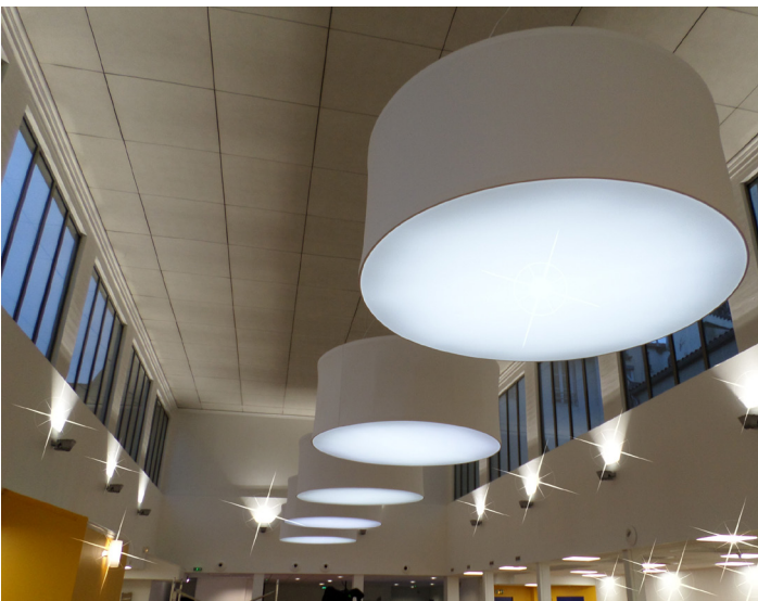
Shopping mall, France. Lights. Dia.:1,90 m. Total thickness 800 mm. Colour and translucent white covering. Integrated lighting.
