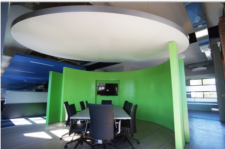
Offices, Greece. Suspended custom frames. Various sizes. Total thickness 280 mm with custom covers. Translucent white covering. Lighting solution.
