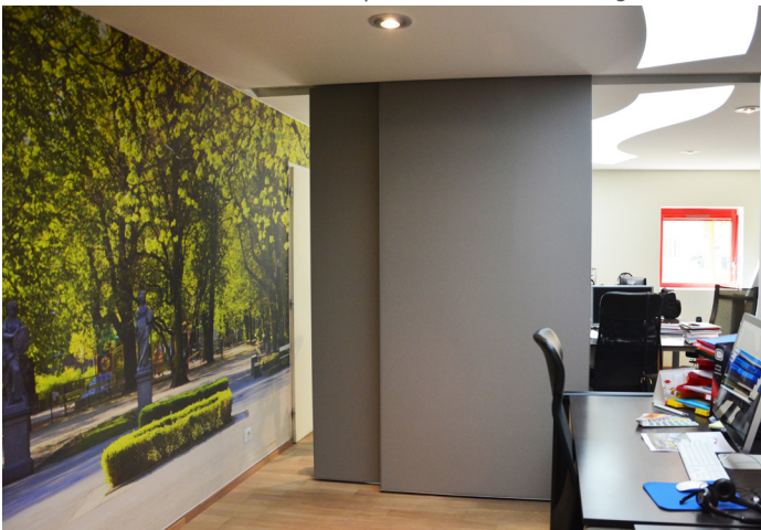
Offices, France. Rail-mounted sliding dividing wall. Dim: 1.20 m x 2.20 m. Thickness 100 mm. Acoustic absorption and colour covering.
