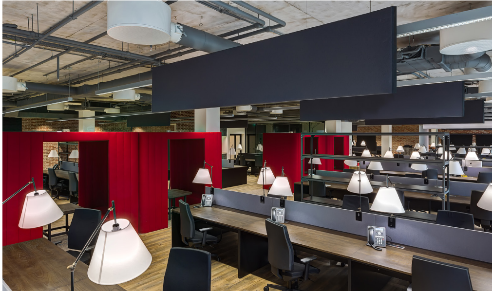
Classroom, USA. Acoustic baffles. Dim.: 0,60 m x 2,80 m. Acoustic absorption and colour covering.
