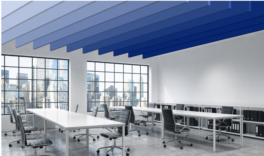
Classroom, USA. Acoustic baffles. Dim.: 0,60 m x 2,80 m. Acoustic absorption and colour covering.
