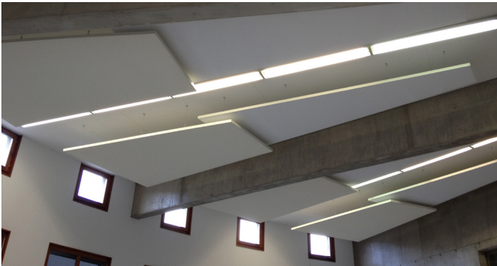
Multi-function room, France. Trapezoid acoustic frames. Different dimensions. Thickness 43 mm. Sound absorption and covering.
