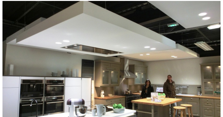
Store, France. Rectangular acoustic frames. Dim: 3.20 m x 1.80 m. Thickness 140 mm. Sound absorbent and white finish. Integrated light and hood.
